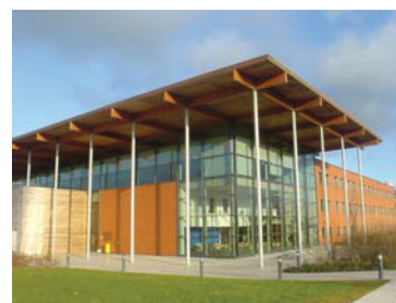
Cambridge Gates Building
